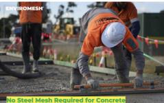
Concrete is Reinforced with Synthetic Fibres
