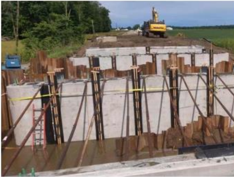
Precast piers, UHPC2.0™ connections
