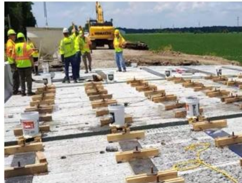
Precast bridge decks, UHPC2.0™ connections
