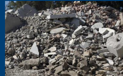
Construction wastes demolition
